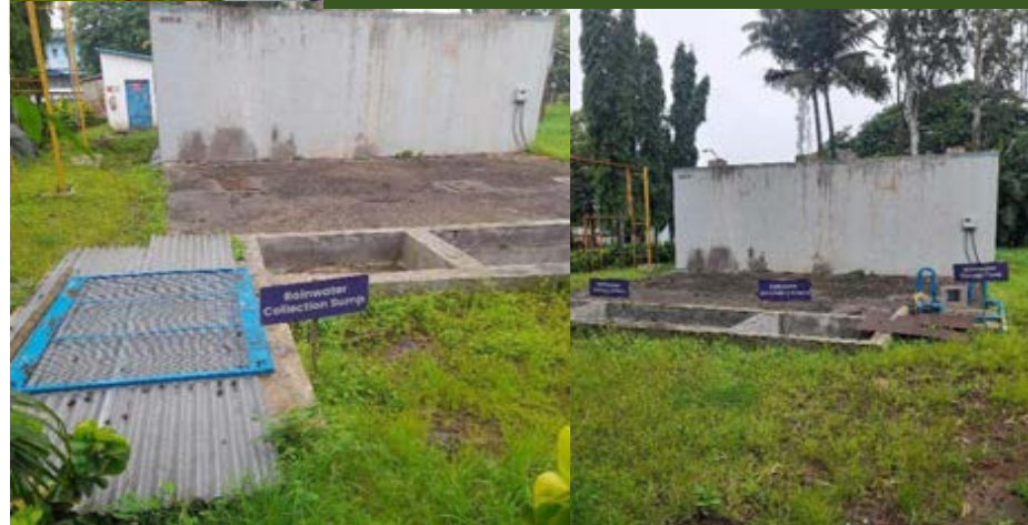
Talegaon: Modular Rainwater Harvesting
